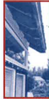
Open eaves, vents not screened (6 pts)
