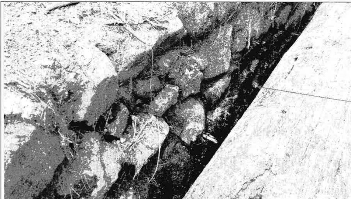
Active Water Leakage Through the Masonry Stone
