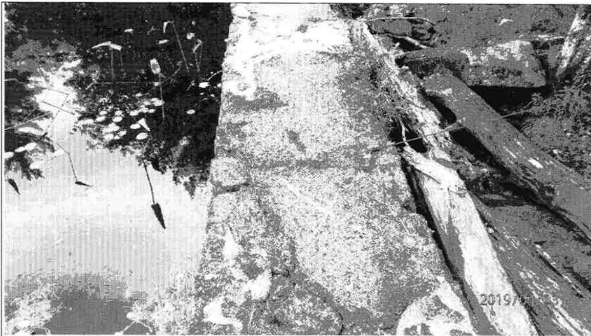
Delamination on Crest
