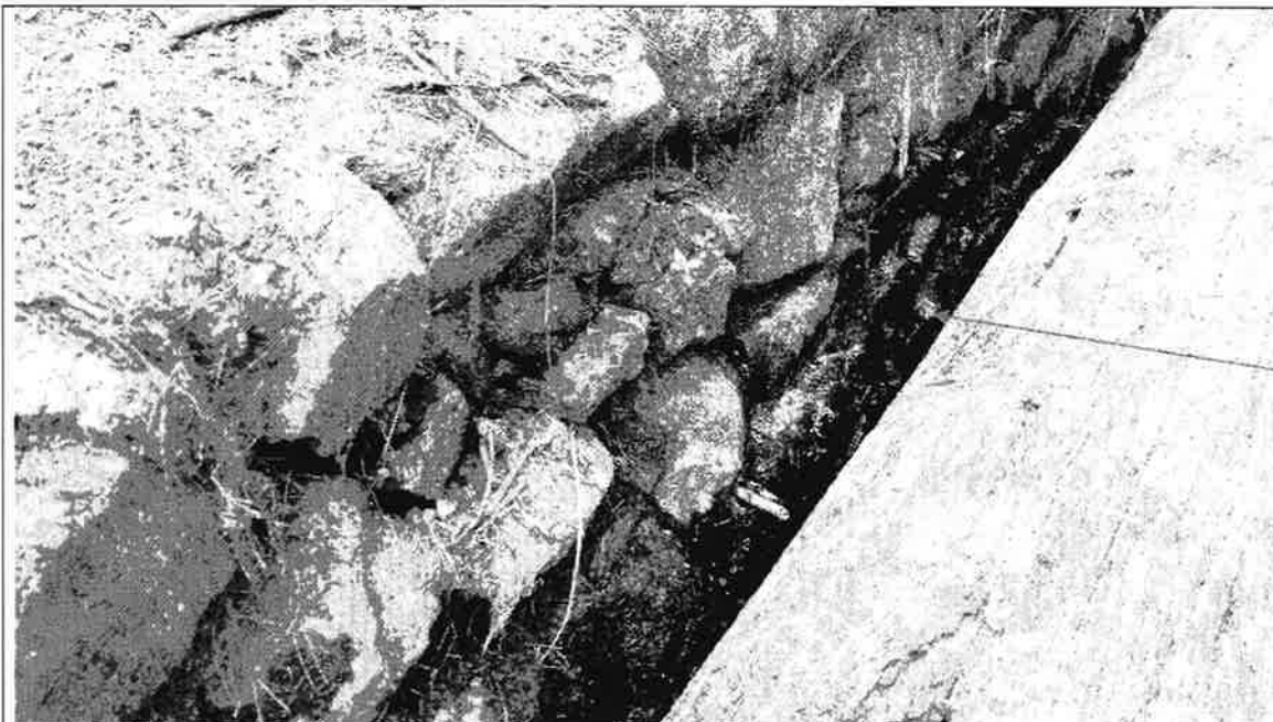
Active Water Leakage Through the Masonry Stone
