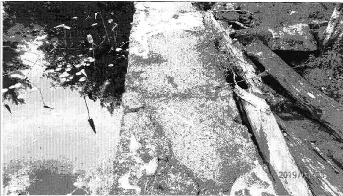
Delamination on Crest
