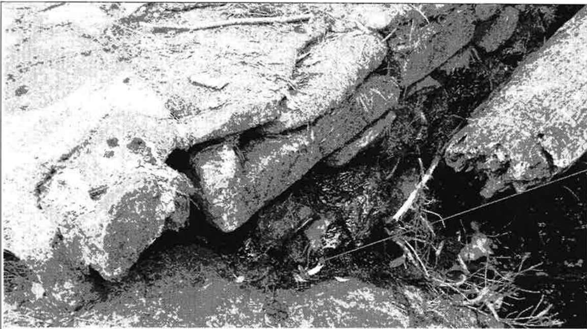
Active Water Leakage Between the Masonry Stone and Bedrock
